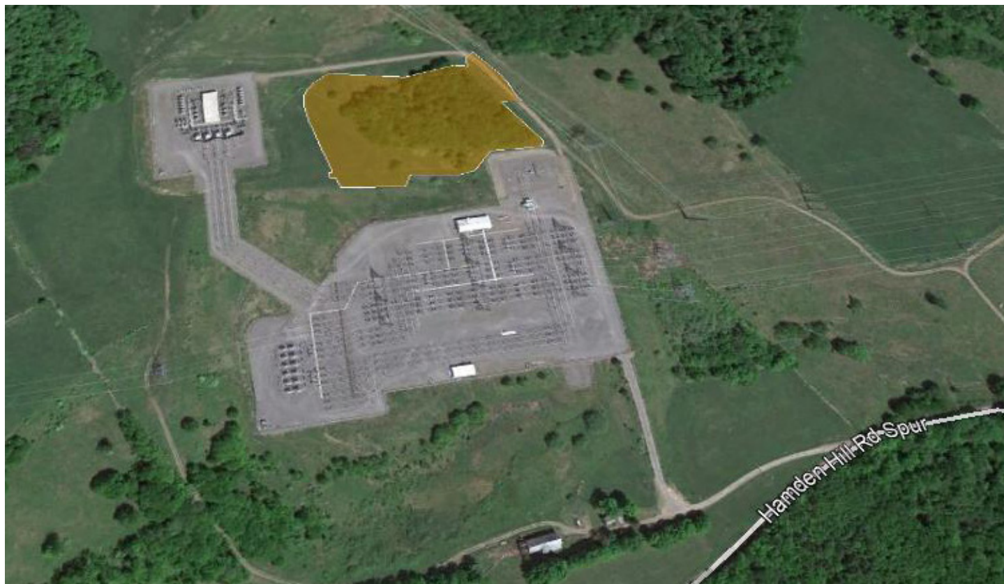
Figure 1: Proposed location of Fraser Substation Expansion (orange) adjacent to NYSEG's existing Fraser Substation facilities.
