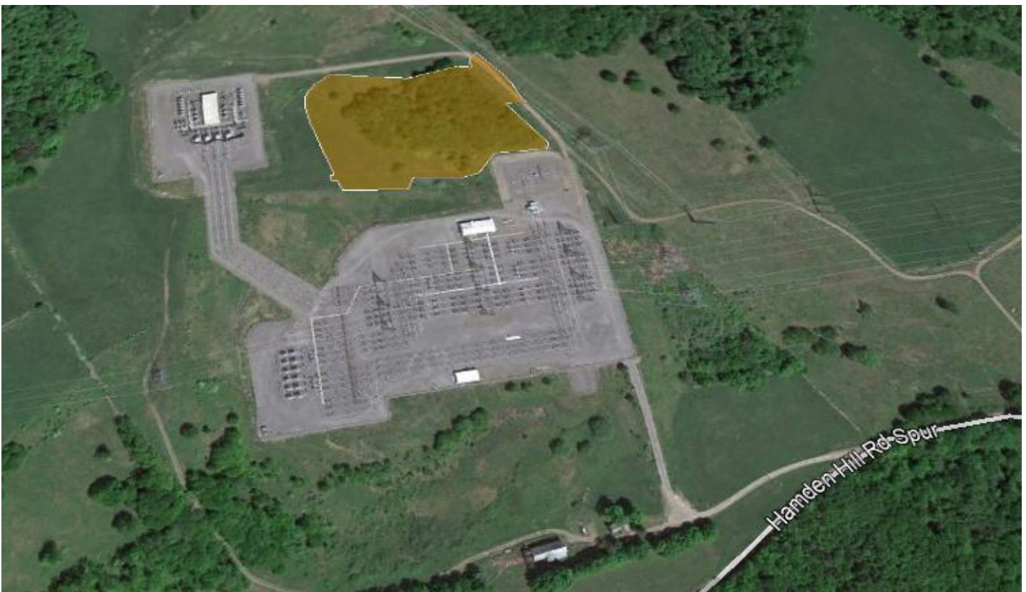
Figure 1: Location of Fraser Substation Expansion (orange) adjacent to NYSEG's existing Fraser Substation facilities.
